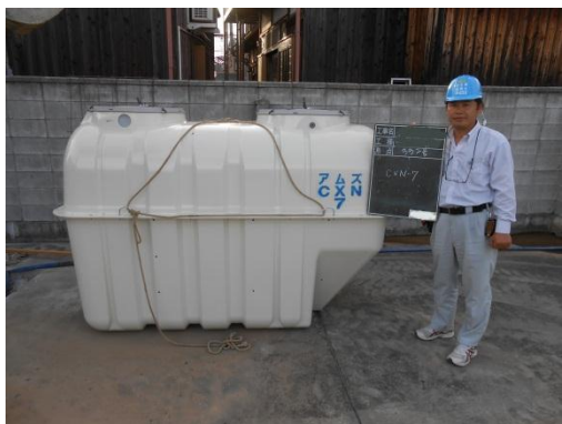
NO.7 浄化槽本体搬入
